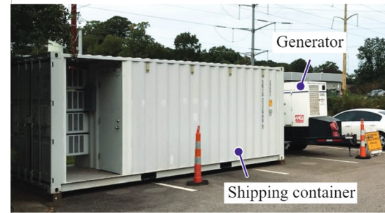
MUSE SST system container system Internal dimensions: 4.4 m x 2.33 m x 2.33 m
